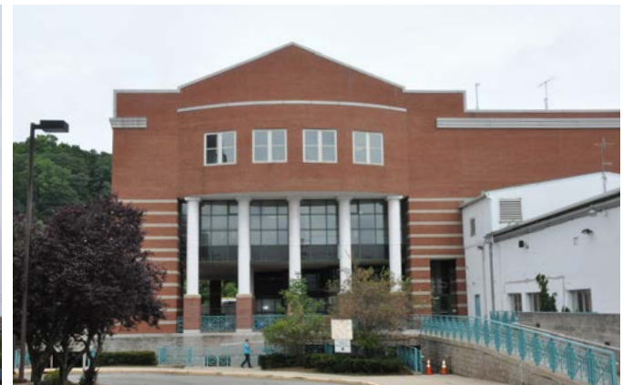
The Sussex County Judicial Center in Newton as it appears today.
